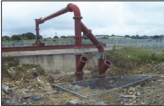
Figure 7a Pump Installation 2001
