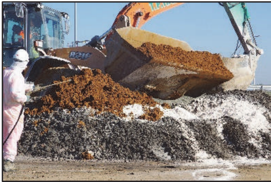
Figure 13a Incorporating HFO with contaminated soils
