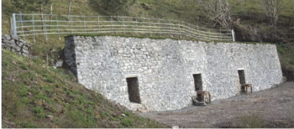
Figure 8: Restoration of the Ecton Mine dressing floor wall following detailed archaeological investigations, as restored in 2016 with financial support from Historic England
